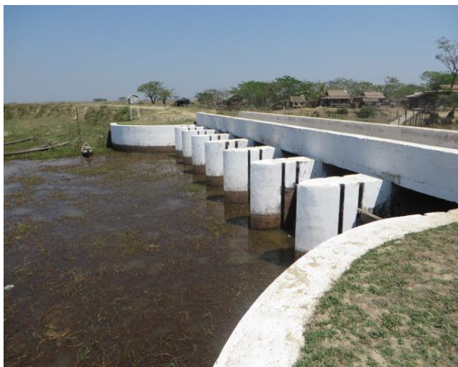
Sluice gate for irrigation water
