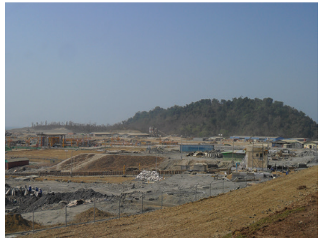
Oil and gas terminal in construction
